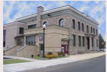
Downingtown Main at Lincoln and Brandywine Avenues has been the headquarters location for DNB First for most of the Bank's existence.
